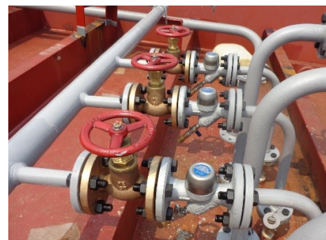
RL 500PF applied on live steam pipes
