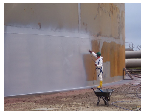
Applying RL 500PF on large tank externals
